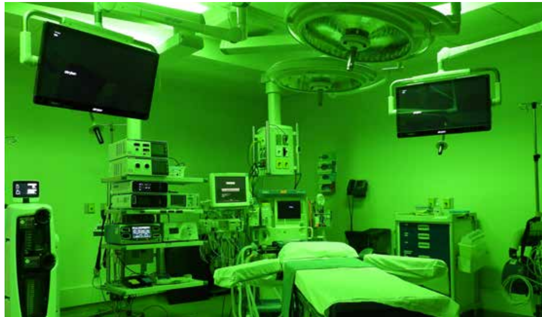
One of the Regina General Hospital operating rooms in full surgical lighting. Green lighting is used to provide adequate ambient light and increased blood contrast, reducing eye strain for the surgical team
